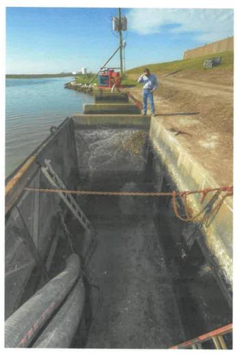
Engineer Steve Matula inspects the removal of dirt and debris from the exit gate May 15 at the Velasco Drainage District's East Levee Pump Station.
