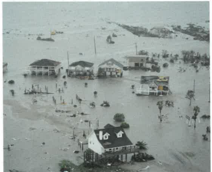
Bolivar Peninsula following Hurricane Ike, 2008.
